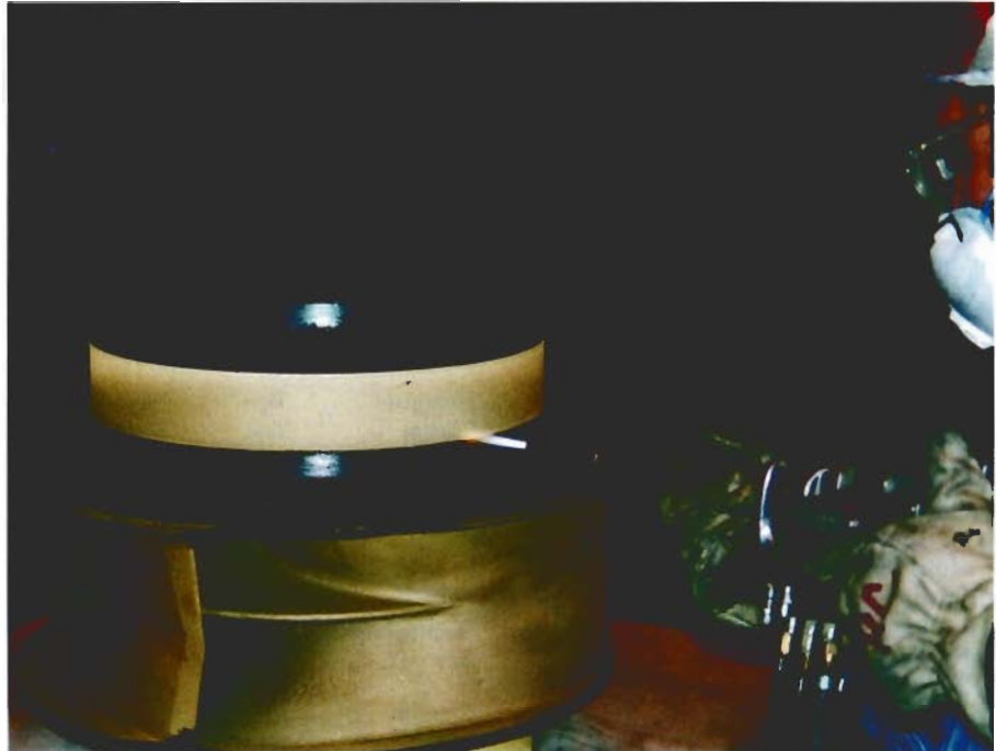
Fig. 3 — A craftsman rebuilds a ring section of an impeller by flame spraying it with a bronze coating, which will be machined to its final dimensions.
